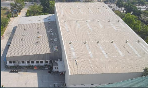
Corporate Office Accurate House, 78/1, Dangat Industrial Estate, Shivane, Pune-411023
